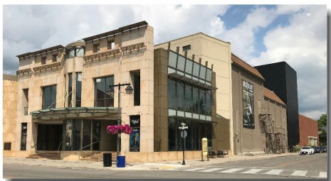
The Avon Theatre - which features a proscenium stage - on Downie Street in downtown Stratford. The Studio Theatre - which features a thrust stage - is visible on the right (back of building). Jaan PILL photo
